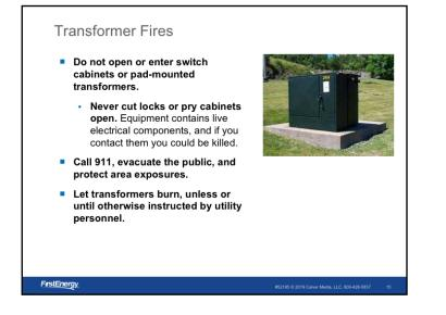
Transformer fires. Burning transformers call for similar procedures as substation fires.
